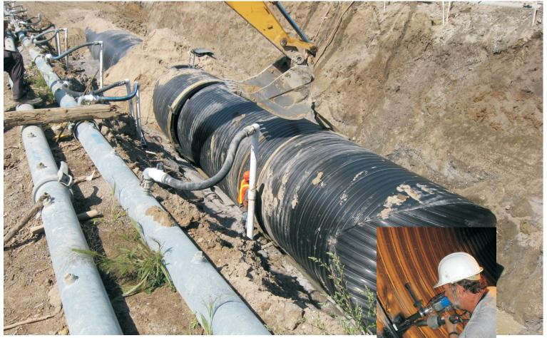
An extensive stormwater storage system was recently installed beneath a sports field at a High School in Unionville, Ontario. The stormwater system collects the rainwater during wet weather and uses the captured water to irrigate the sports fields during dry periods.
